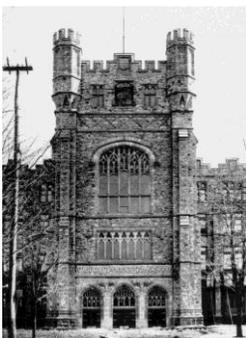
**Reflecting the Past:** The original tower was intended to be the focal point of the building. Regrettably, the tower had to be removed by 1916 because unstable soil conditions would not support its massive weight. Nearly 100 years later, the architects created the new lantern that not only evokes the spirit of Ewart’s early tower, but also encloses a new butterfly staircase and heralds the 21<sup>st</sup> century transformation of the museum. Image from Library and Archives Canada.
