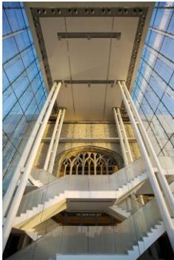
**Innovative Engineering Solution:** Unlike David Ewart's original heavy tower, the new structure does not impose any weight on the existing masonry walls. The Queens' Lantern actually hangs from a specially constructed roof that is cantilevered from concrete walls for the new elevator shafts inside the building. Four large steel columns provide the structural support for the roof, from which hang the panes of glass that form a transparent box.
